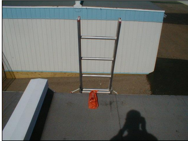
Ladder tied-off with rungs well above roof
