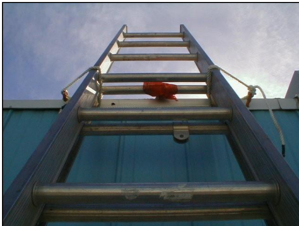
Ladder tied-off with rungs well above roof
