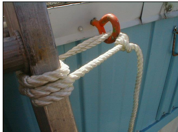
Ladder tied-off with rungs well above roof
