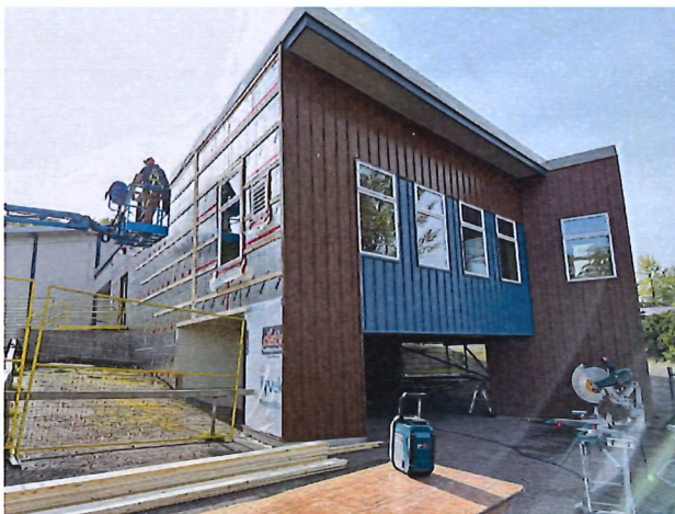
Telkwa Elementary building envelope install
